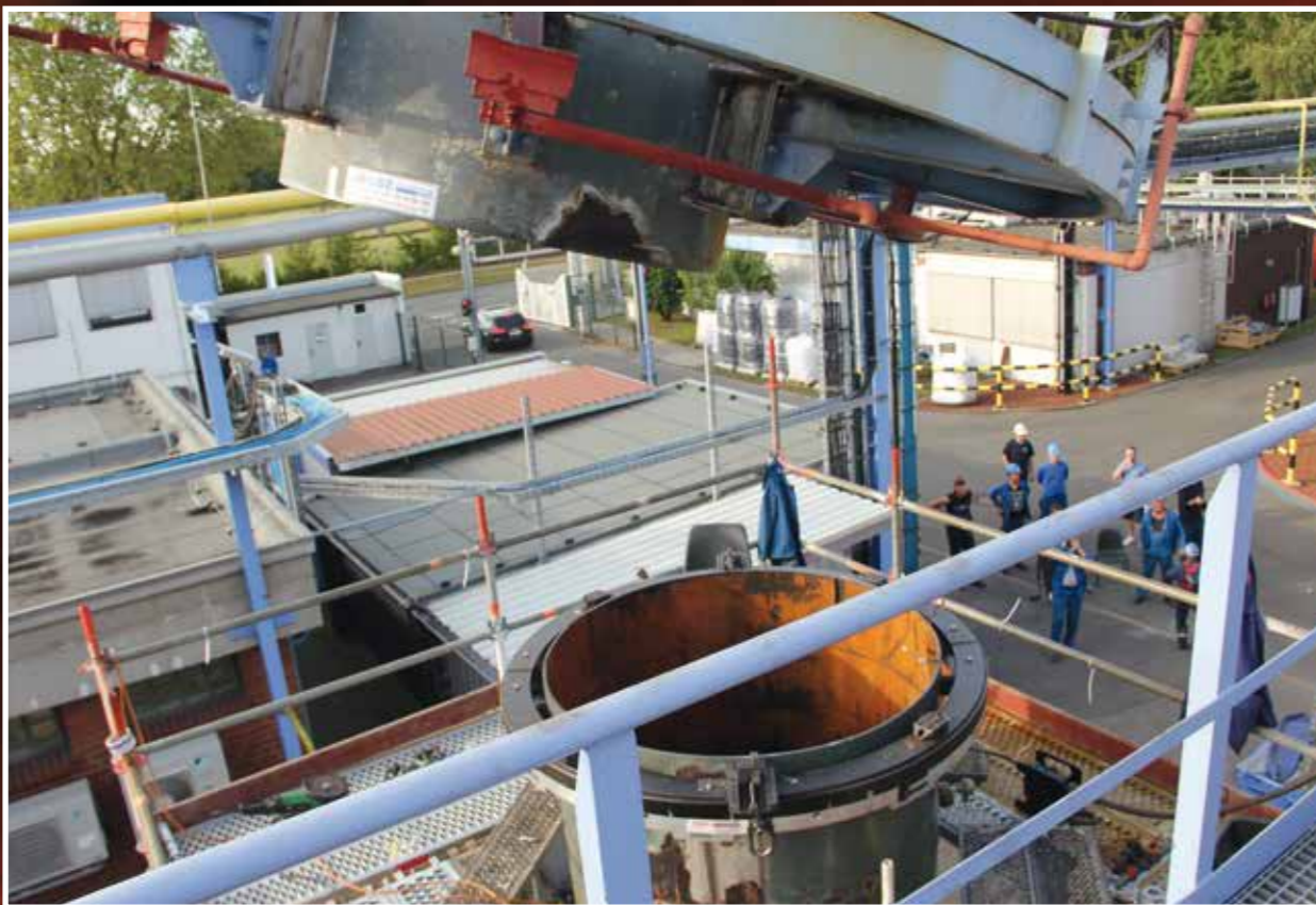
Disassembly of the column head – cutting, bevelling and preheating at a height of 40 meters.
