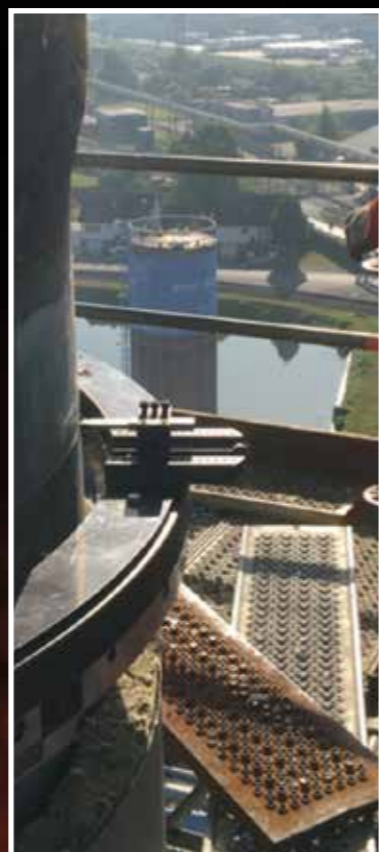
Disassembly of the column head – cutting, bevelling and preheating at a height of 40 meters.
